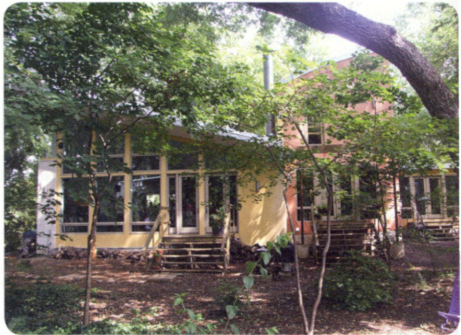
Passive solar design ICFs, SIPs, and energy-efficient equipment earned this Dallas home a high HERS rating.
